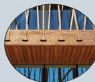
IN THE SLABS- MITERED BUTT JOINTS ARE USED.
